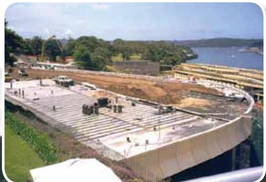
The Eastern Distributor is representing a massive project in Sydney that includes a massive concrete overpass with a green roof above Cahill highway. For the project, 7000 m<sup>2</sup> of Atlantis® Flo-Cell® drainage cells were used to protect and improve the permeability of the hydrological system.
